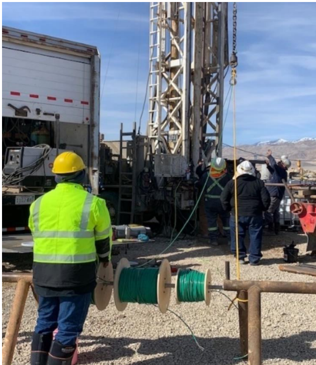
Photograph, southwest view of DH-1 drill-site. Showing DH-1A VWP installation.
